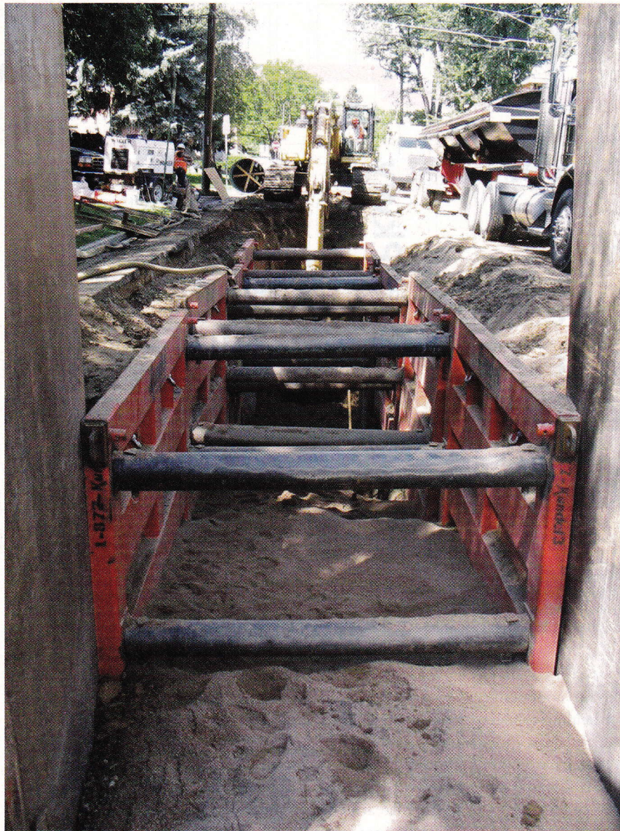
A 54 in. (1,350 mm) diameter conduit was installed in one of Denver's older residential neighborhoods. Narrow streets and the presence of many utilities and trees made for difficult conditions.
