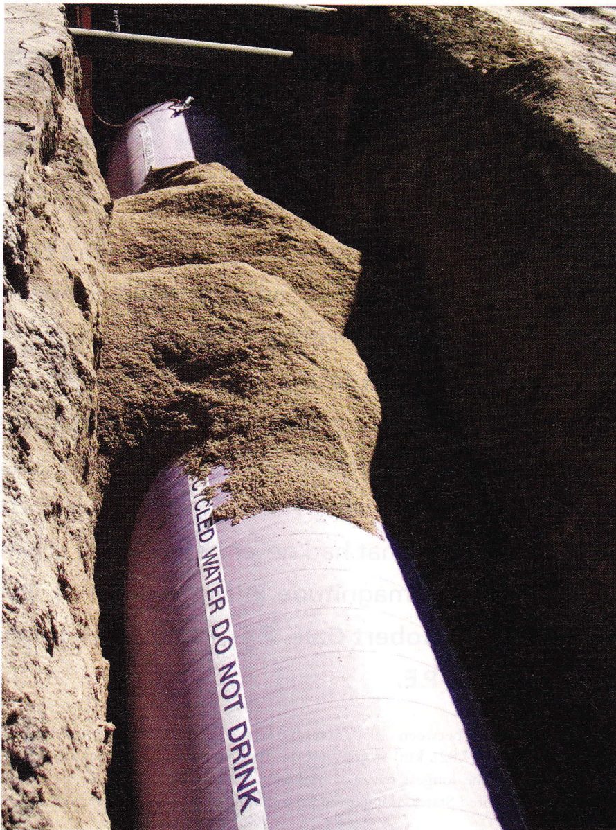
To distinguish them from drinking water and sanitary sewer pipelines, the pipelines for recycled water pipelines, as well as the manhole covers above them, were required to have a purple exterior. Two sides of each pipeline were required to carry the warning Recycled Water—Do Not Drink.
