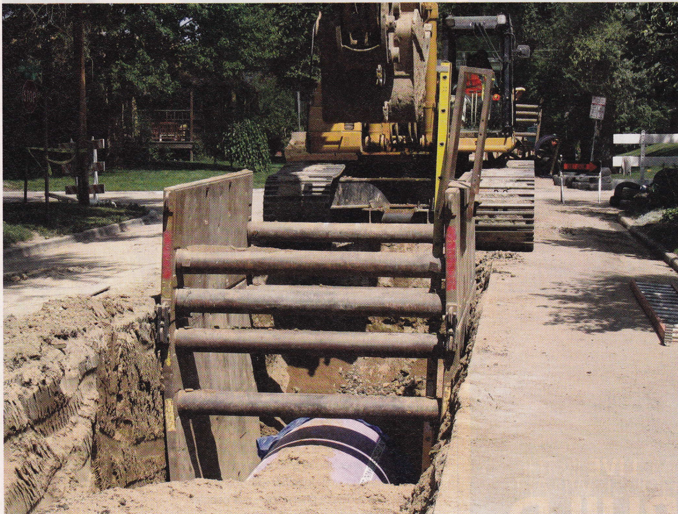
The area between the new reservoir and the pump station primarily consists of gridlike residential blocks and offered hundreds of potential alignments for the conduit. The area's narrow residential streets, which typically are 30 to 36 ft (9.1 to 11 m) wide from curb to curb, provided an obvious solution, as they enabled Denver Water to construct the pipeline in areas with less traffic.
